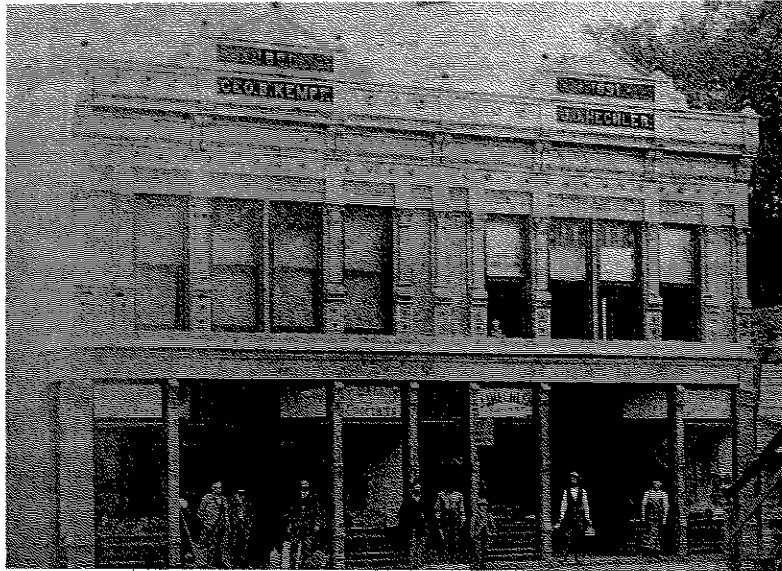
First Hechler and Kemp building, 1891.
